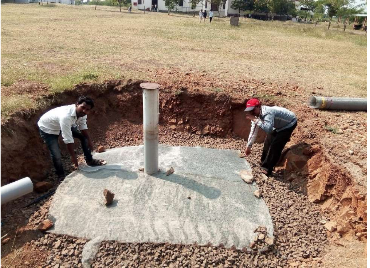
Fig4: Placing layer of filter bed
