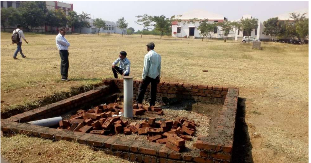
Fig.5: Principal sir observing construction of brick side wall
